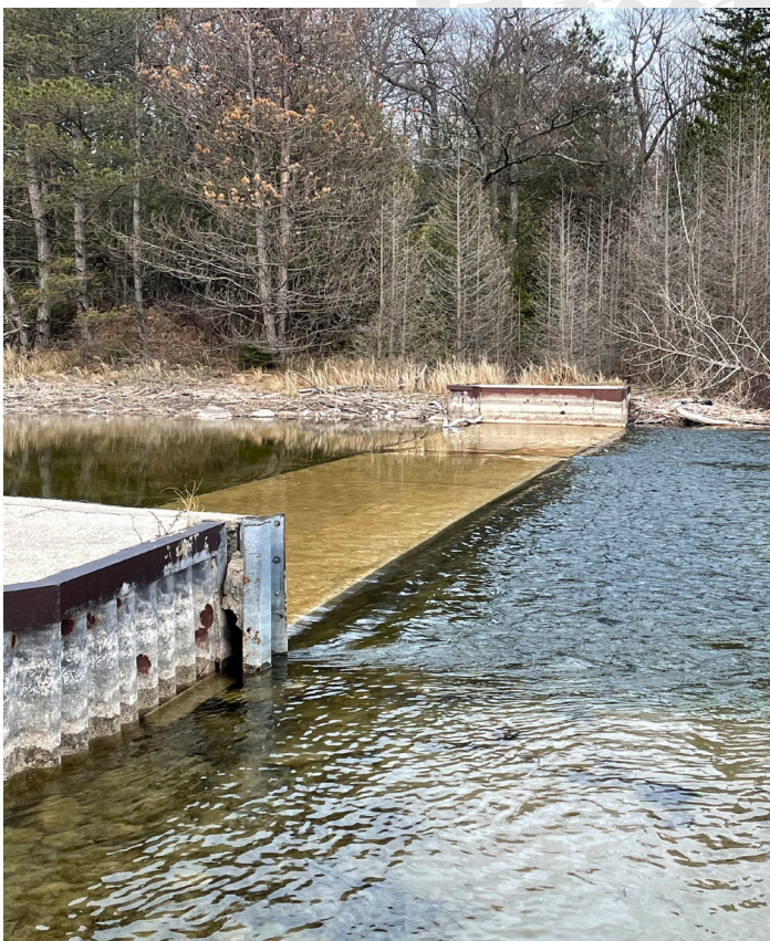
Check out the drop over the Dam
